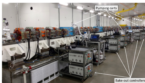
Figure 4: A storage ring arc ready for the bake-out process.
