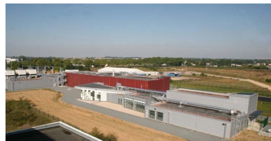
Figure 4: Completion of the accelerator building (October 2014). The beam axis is 8 meters underground.
