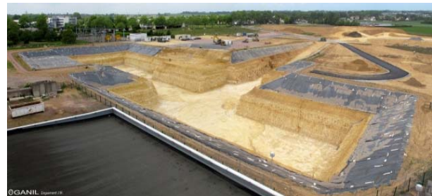
Figure 2: End of excavation work mid 2011.
