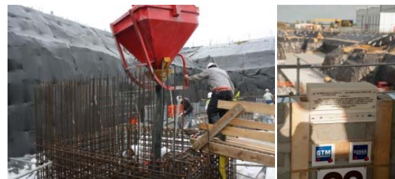
Figure 3: First concrete in September 2011 and the foundation stone ceremony in October 2011.
