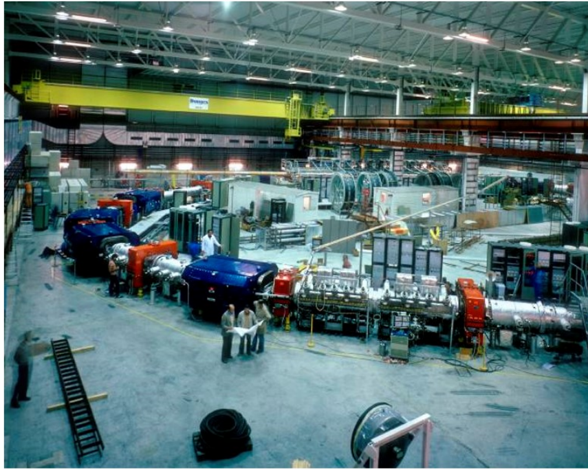
Figure 6. View of the Antiproton Accumulator during construction.
