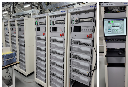
Figure 8: SSPAs installed for the SRF cryomodule test.
