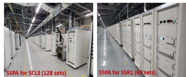
Figure 3: SSPAs for SCL3(left) and SSPAs for SSR1(right) installed in each gallery.
