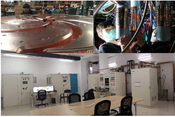
Figure 6: Installation of RF cavities (upper left), coaxial lines (upper right) and RF amplifiers (lower).
