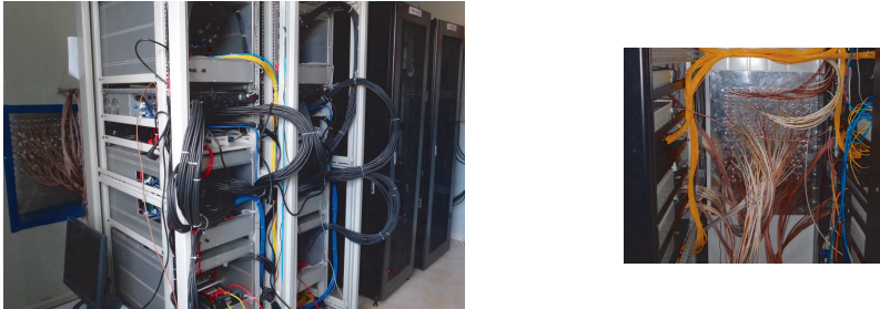
Figure 4 – Digital system(Left) and bulkhead connectors between analog and digital system(Right).
