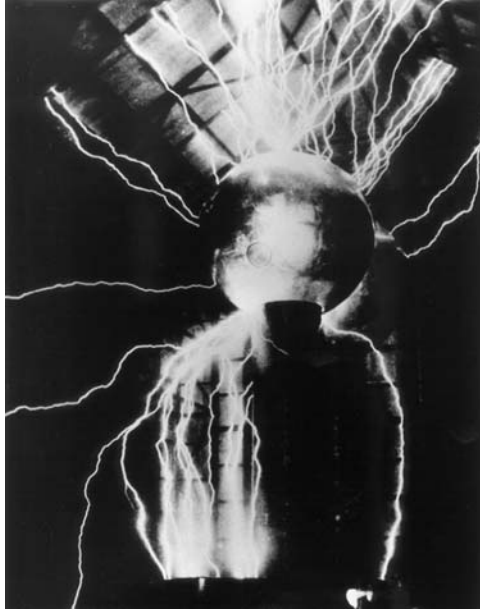
Fig. 5.2. Van de Graaff’s twin-column electrostatic accelerator sparking to the roof and the walls in the Round Hill hangar in Connecticut in 1932 (Reprinted from [2], copyright (1974) with permission from Elsevier)
