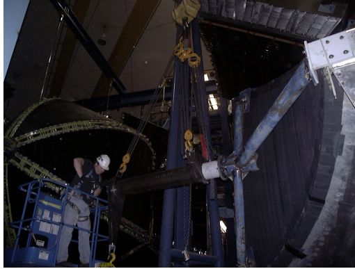
Figure 5.21: Photograph of one of the six Cherenkov Counter sectors during installation in the CLAS detector. The drift chambers are shown in the background on the left of the photograph [97].
