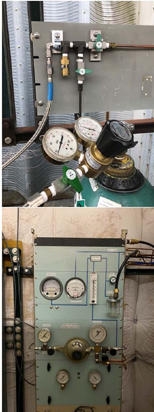
Figure C.22: Pictures of the cylinder and setup outside MC7 and the gas panels inside the enclosure.
