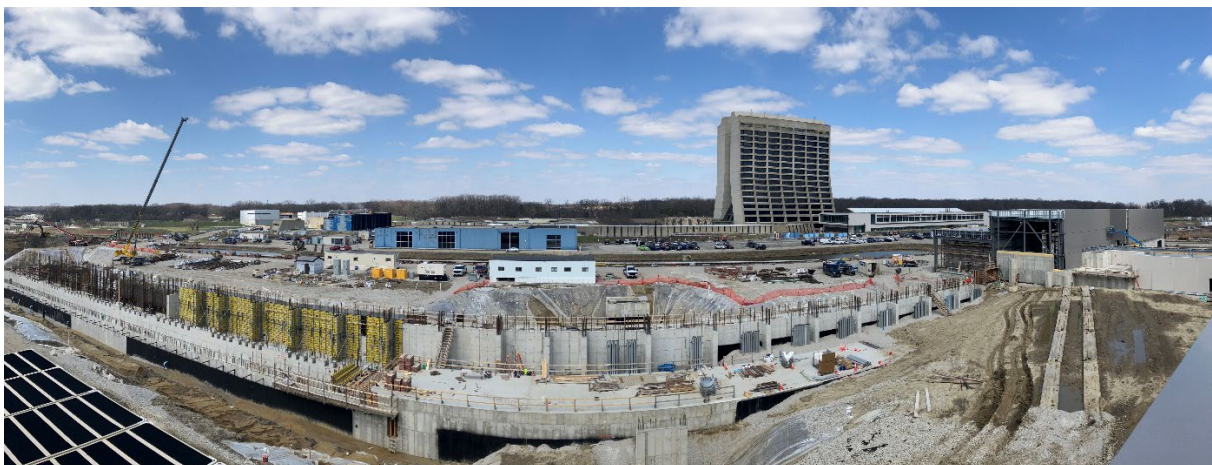
Figure 1. PIP-II construction area (in April, 2025)
