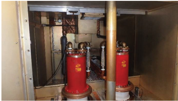
Figure 9: PA2 with stainless steel bellows.
