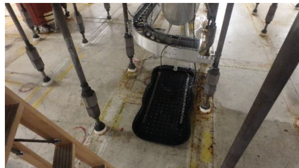
Figure 12: Photo of water leak sensors tray.
