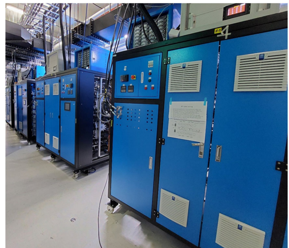
Figure 2: The 320 kW solid-state power amplifier racks.
