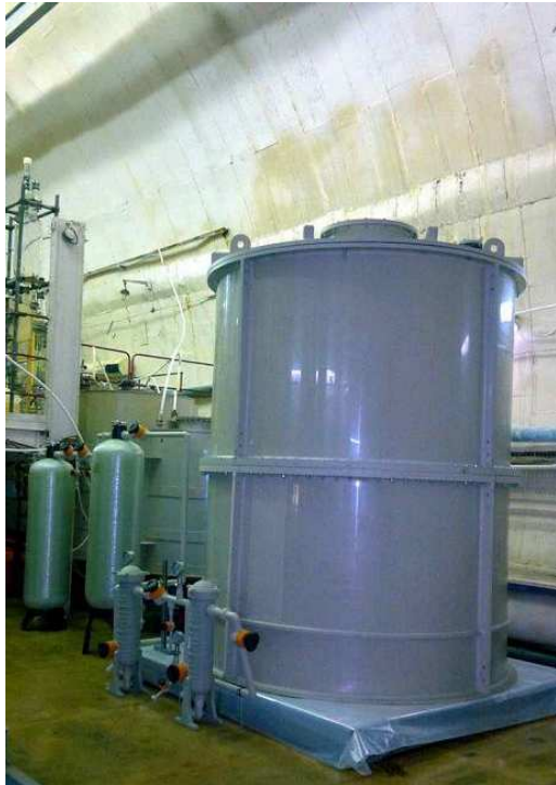
Figure 1. External tank from polypropylene.
