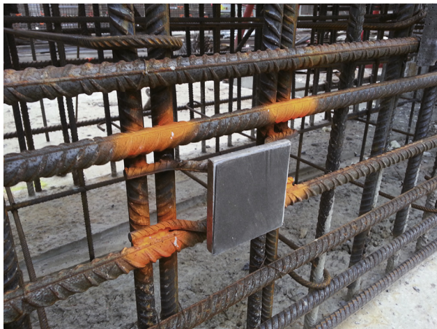
Fig. 41. Iron re-bar earthing mesh within the concrete walls, floor and ceiling of ELI Beamlines experimental facility. A grounding plate is also shown.
