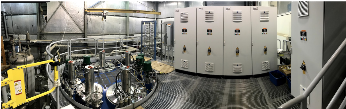
Figure 3. Panoramic photograph of the SC1R subatmospheric cold box installation showing the top of the cold box and cold compressors (left) and variable frequency drives and active magnetic bearing controllers (right).
