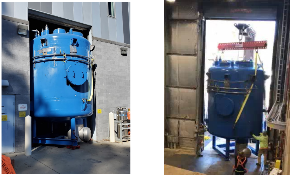
Figure 2. Left: Moving the SC1R 2 K Cold Box assembly out of the workshop on 10 ton machine skates. Right: Moving the cold box into the CHL building using the 60 ton forklift.
