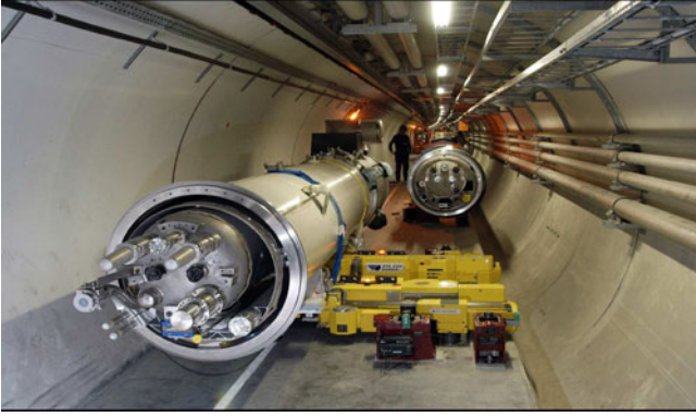
Figure 6. Example for the tight manoeuvring in the LHC tunnel during installation. The picture shows the installation of the low-B triplet magnets near the experimental detectors
