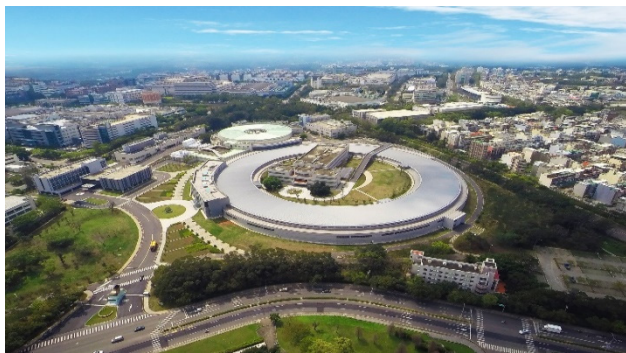
Figure 1: Top view of the TPS facility.
