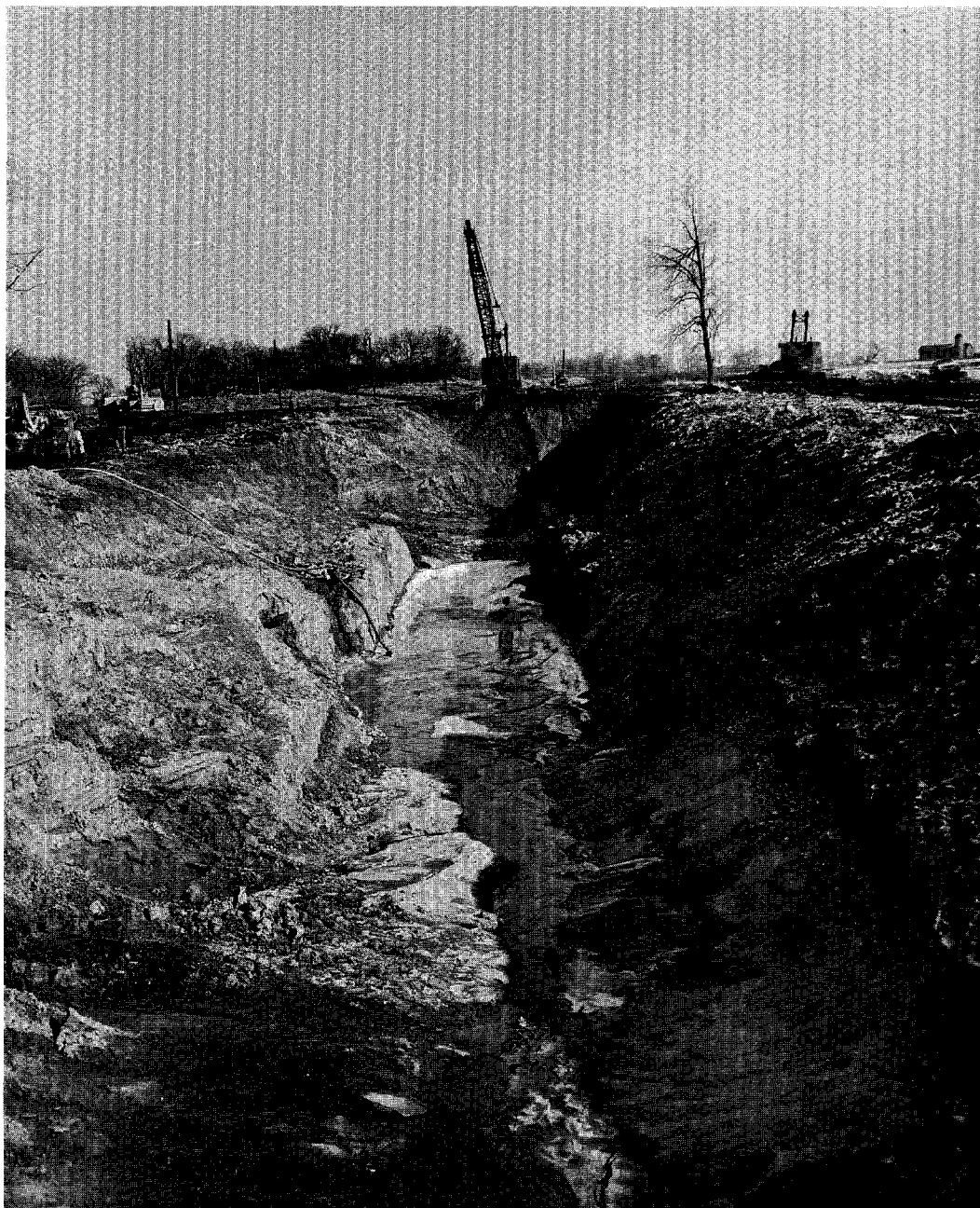
EXCAVATION FOR THE MAIN ACCELERATOR
