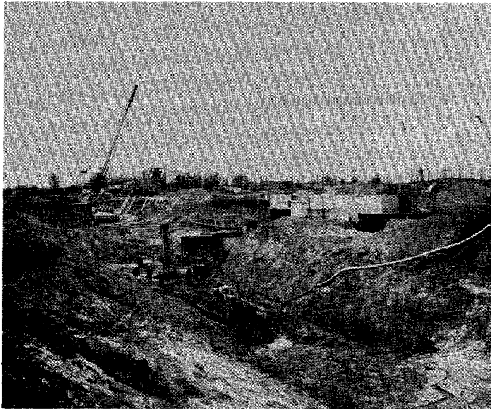
Fig. 4. The Transfer Hall excavation, looking south from the same point as the cover photograph. The Cross Gallery is to the right.
