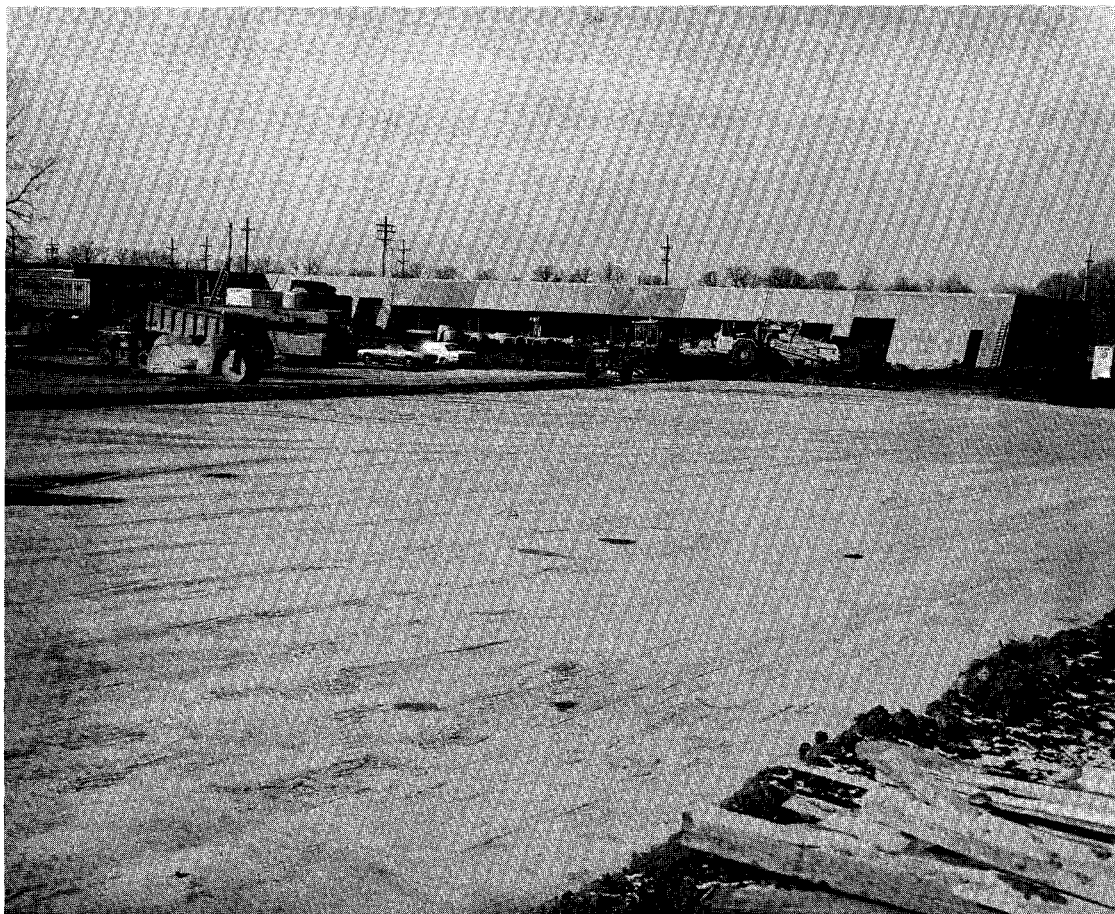
Fig. 1. The Linac Building. The photograph was taken from what will be the front of the Central Laboratory. Grading work in the footprint area can be seen in the foreground.
