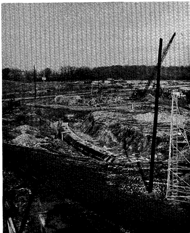
Fig. 2. The Booster Enclosure This photograph was taken from almost the same position as Fig. 1 of last month's report. Just to the left of the crane can be seen some of the wiring and piping conduits that will run between the tunnel and the Booster Gallery above it.
