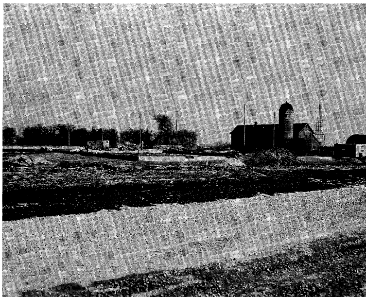
Fig. 5. Foundation work on the Industrial Buildings.
