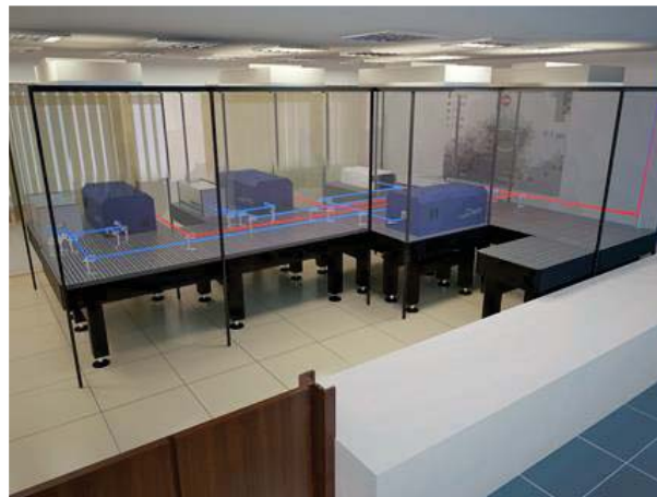
Figure 3. Laser room with installed lasers.
