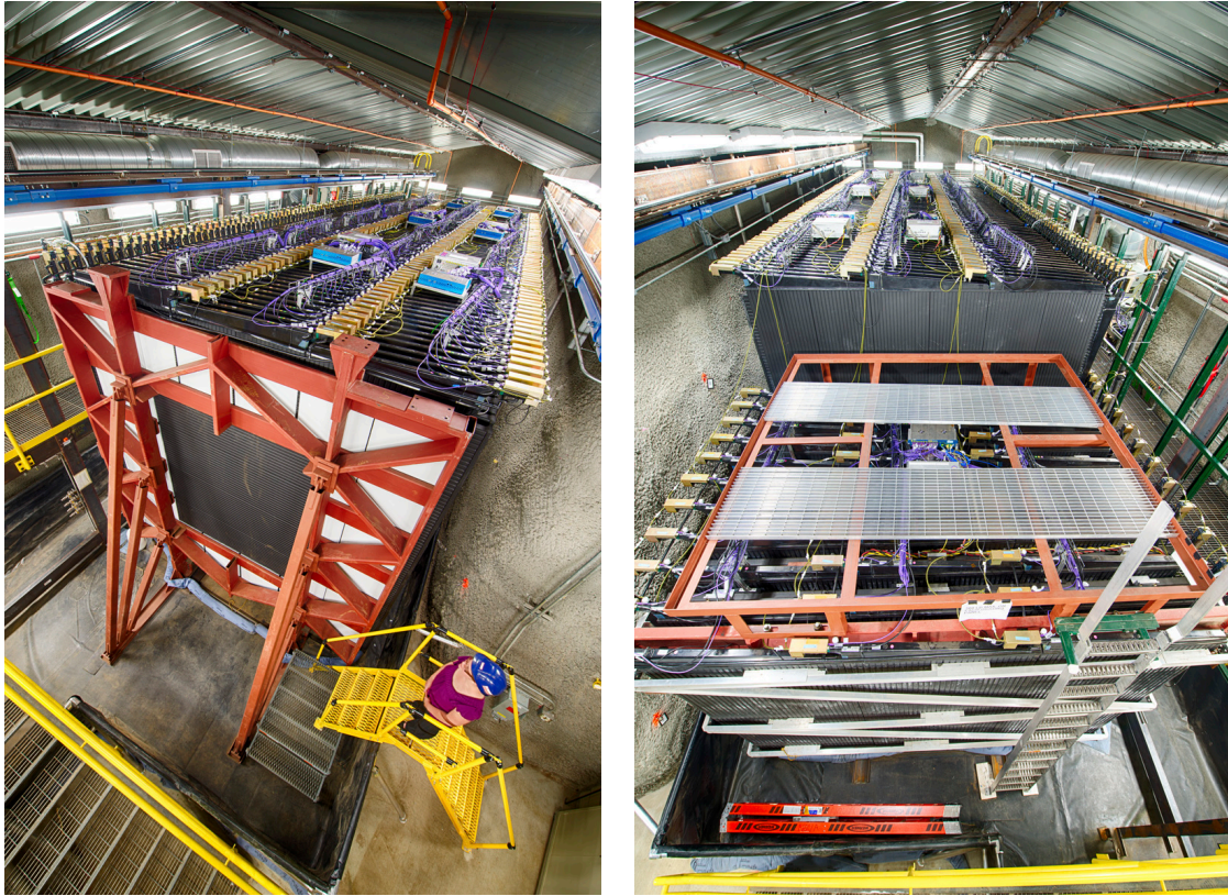
Figure 3.13: The NO \nu A ND. Left: View from the side where the beam enters the detector. The red structure is a bookend and not part of the active detector. A person is seen on the right for scale. Right: View from the side where the beam exits the detector. The red and grey structure above the muon catcher is for worker access to this detector region and not part of the active detector.
