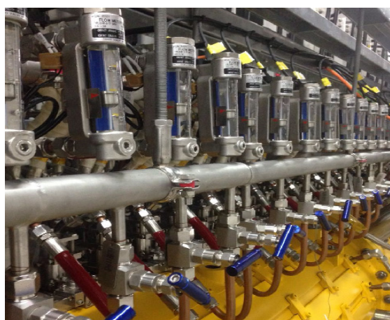
Figure 6: Flow switch placing on the Drift tube cooling channels.
