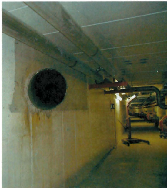
Figure 8: End of carrier pipe where it penetrates the wall of the Main Injector tunnel. This pipe was installed to enclose a low-energy beamline from the Main Injector at MI-10 to the experimental hall at MI-9. The four penetrations on the ceiling also lead to the location of the future MI-9 enclosure.
