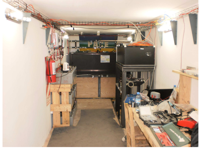
(b) CRLF Core Infrastructure Complete
