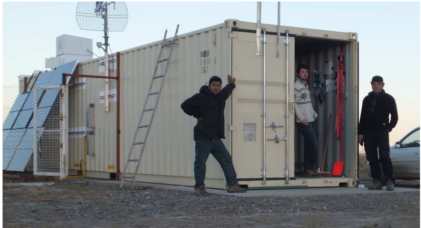
(c) The Outside of the Completed CRLF
