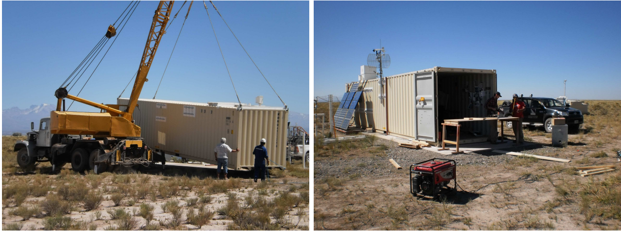
(a) The CRLF Container Being Placed at the CLF Site.
