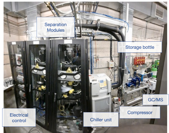
Fig. 1. Picture of the \text{C}_2\text{H}_2\text{F}_4 recuperation system installed at CMS for the RPC detectors.
