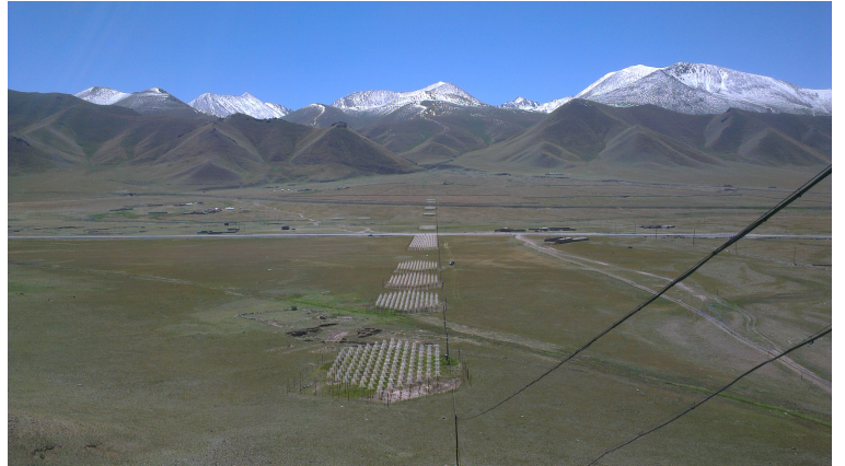
Figure 5.3: Left: layout of the 21CMA experiment, composed of two baselines formed of 40 pods aligned along the East-West and North-South directions. The East-West baseline extends on 2740m, the North-South on 4022m, thus corresponding to equal lengths when projected in the plane tangent to the Earth at the North Pole. The pods are labeled 101 to 120 for the East arm, 121 to 140 for the West arm, 141 to 160 for the South arm, 161 to 180 for the North arm. Pictures of a pod and the Ulaan Observatory buildings are shown in the insets. The Ulaan Observatory buildings, located between the East and West arms of the 21CMA, host the DAQ rooms for the 21CMA and TREND experiments, a mechanical & electronics workshop and leaving quarters. Right: picture of several pods comprising the South arm of the 21CMA. Pods are group of 127 antennas forming an hexagon of 30m length. Also visible at the bottom right corner of the picture is the cable bundle formed by the optical fibers and power supply for the pods.
