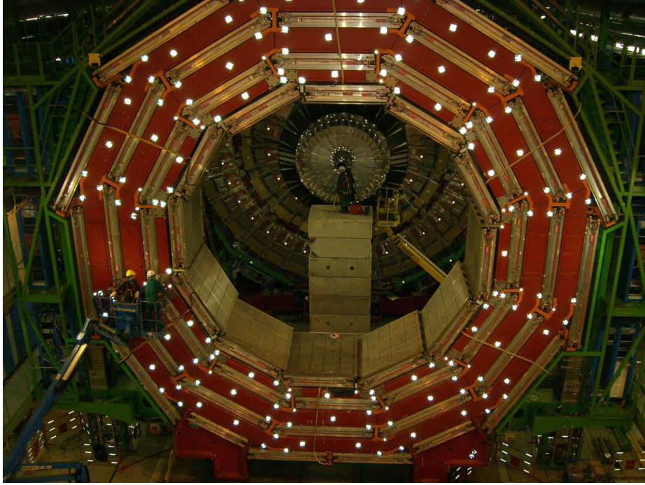
Figure 2-5: A photograph of the CMS detector during the installation phase
