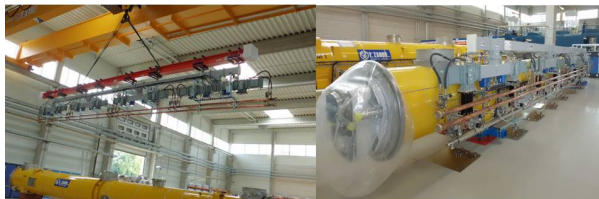
Figure 10: Waveguide installation to module.
