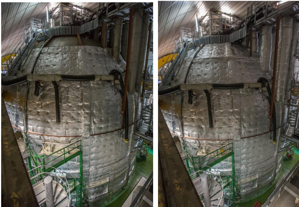
**Fig. 4.14:** Pictures of the Borexino detector water tank covered with the insulation layer, partially in the left picture, and totally in the right one.
