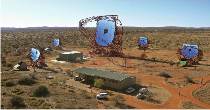
Fig. 5.5 The H.E.S.S. array of IACTs. The medium telescopes CT1-4 are visible at the corners of the array. The large telescope CT5 is at the center. Figure extracted from H.E.S.S. Collaboration (2002)
