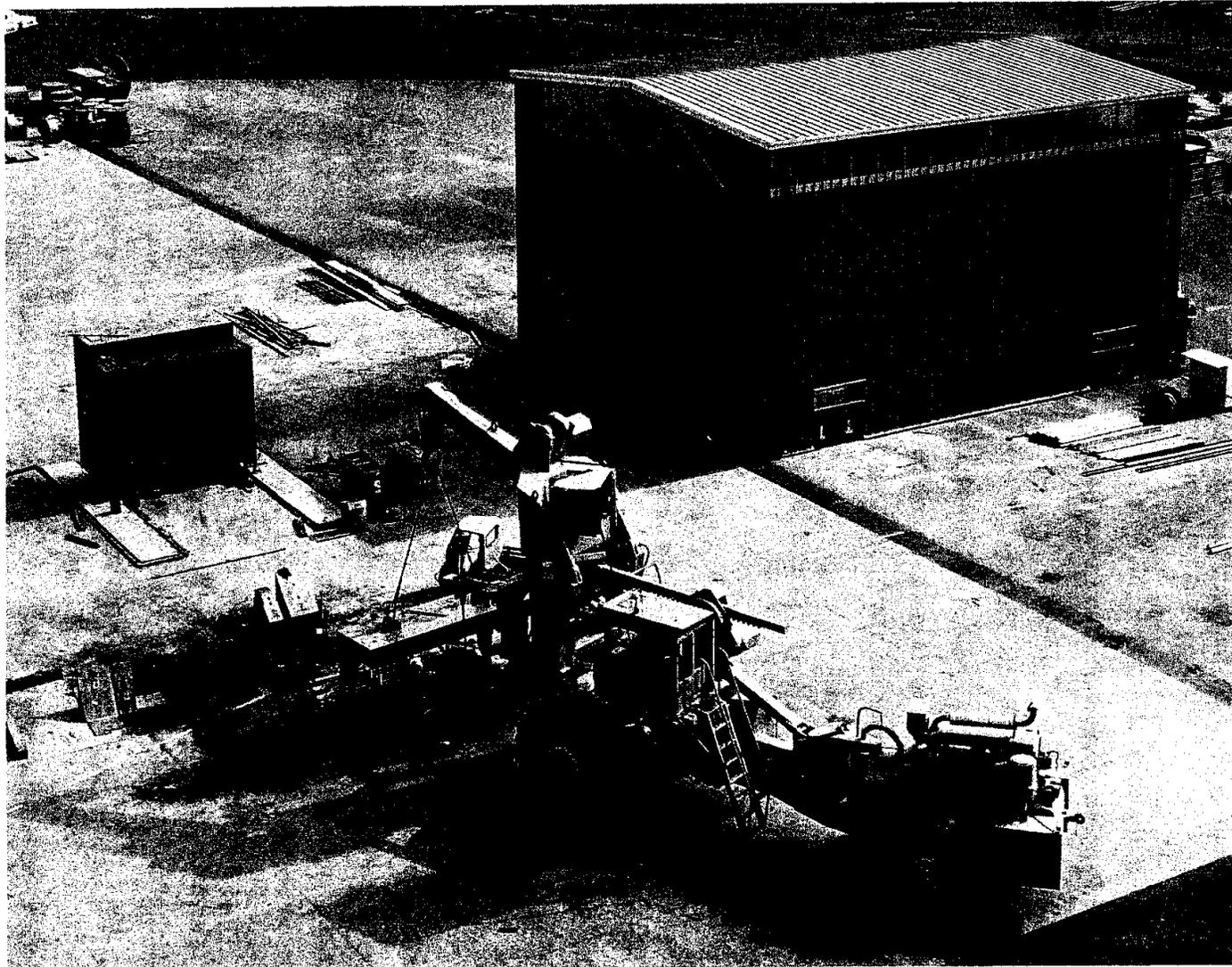
FIG.17-ENCLOSURE AND CRANE FOR 40-INCH HYDROGEN BUBBLE CHAMBER
