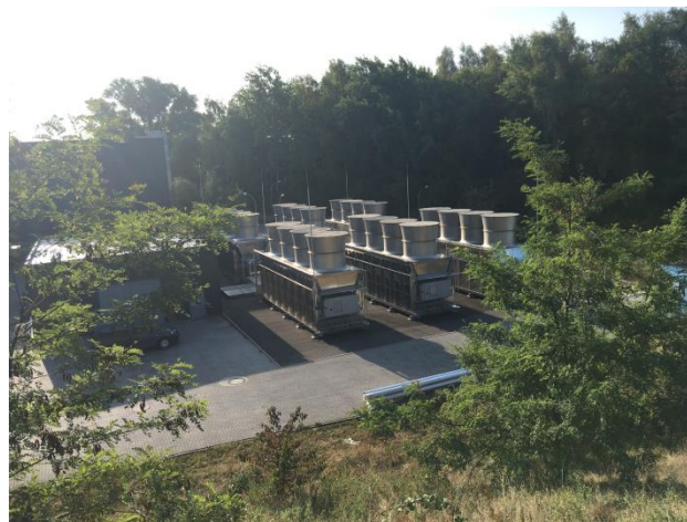
Figure 4: XHM cooling towers for dry and wet cooling.
