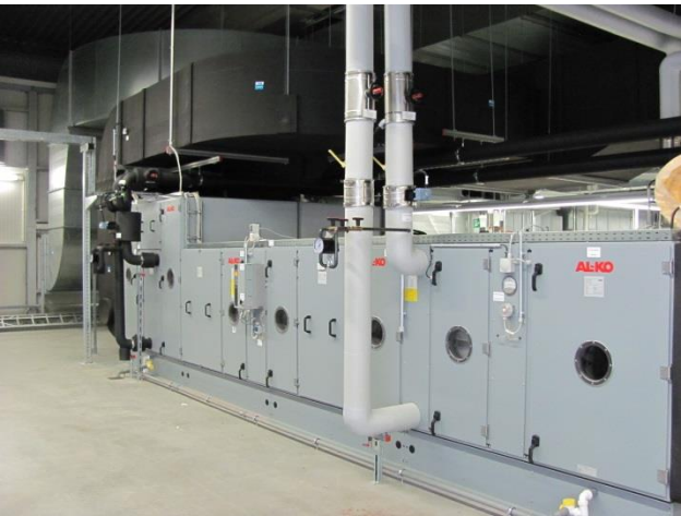
Figure 9: Tunnel Air Handling Unit.
