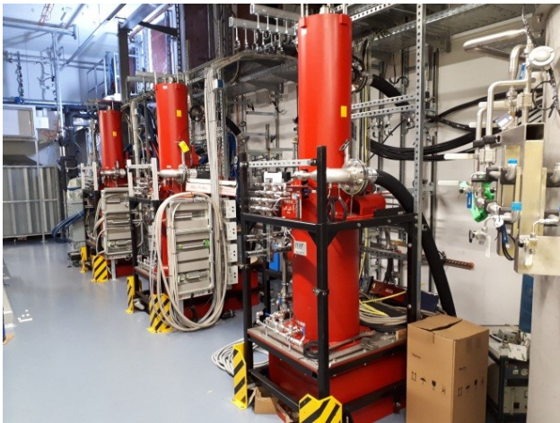
Figure 3: Installed klystrons.
