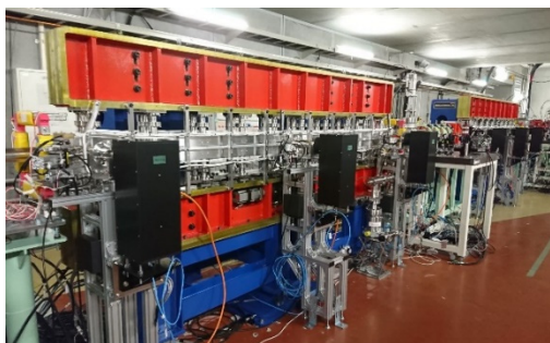
Figure 2: Fixed gap planar undulators installed in the cERL.
