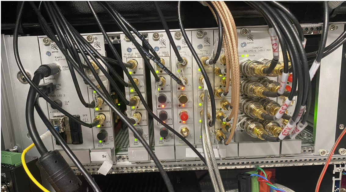
Figure 3.14: ARTIQ crate configuration used to control the 689 nm laser system AOMs. The setup includes a Kasli seed controller (which provides sequence timing control), Urukul AD9910 Direct Digital Synthesizers (DDS) boards for generating RF signals to drive AOMs, Mirny (PLL/VCO-based microwave frequency synthesiser) modules, and a Sampler (analog-to-digital converter (ADC)) module used to digitise analog signals.
