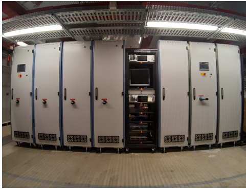
Figure 1: Photograph of the 74 kW (left) and the 56 kW (right) MAMBO SSPA at the electronics area. The middle rack houses two Raspberry Pi based interlock units and a PC as local user interface.
