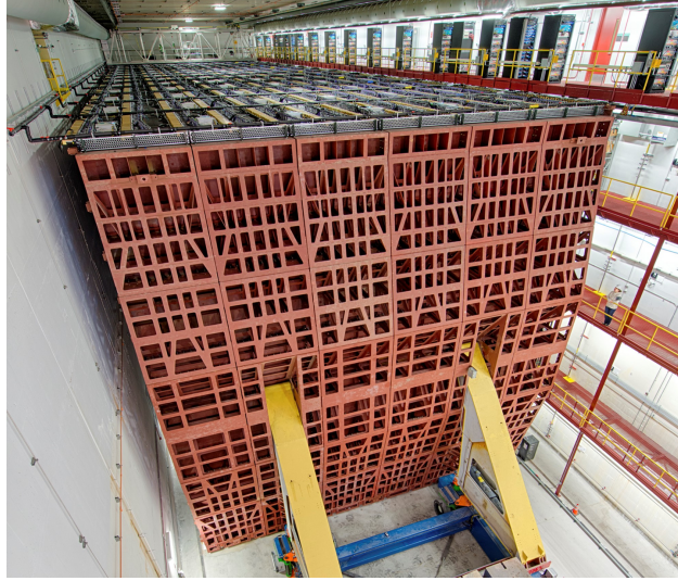
Figure 3.5: A picture of the NOvA Far Detector. Prominent in the foreground is the device used to tilt the planes into place during construction, now used as a structural support. Some of the readout electronics are visible on top. The walking surface of the top floor is roughly at grade.
