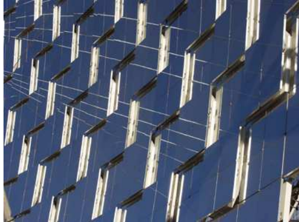
Figure 4.9: Photograph of the chess board assembling of the panels at MAGIC telescope dish.
