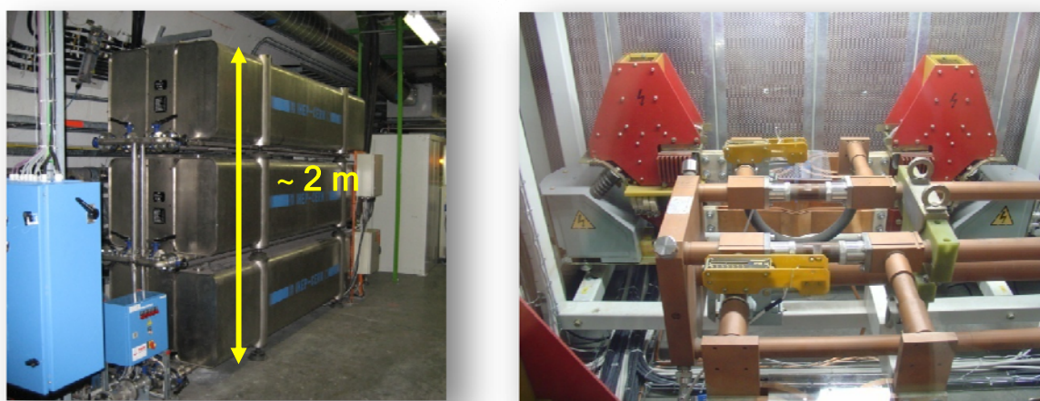
Figure 3.5 _ Dumping resistors for the main dipole magnets (left) and detail of the switches (right).
