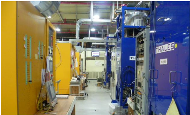
Figure 2: Three 300kW klystrons and KSUs.
