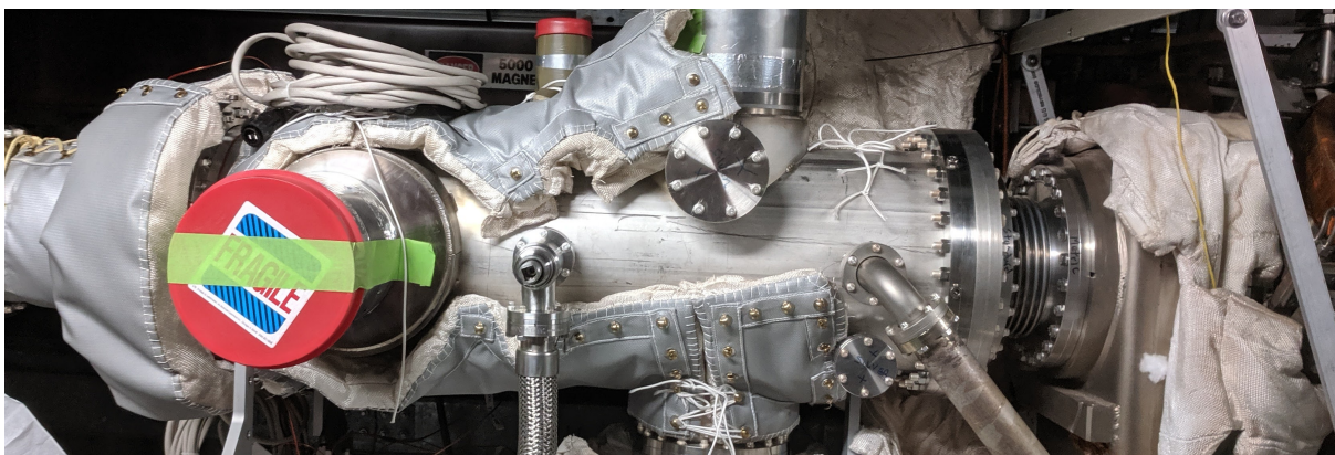
Figure 3.5: Magnet vacuum chamber after installation in ring as it is being prepared for a vacuum bakeout.
