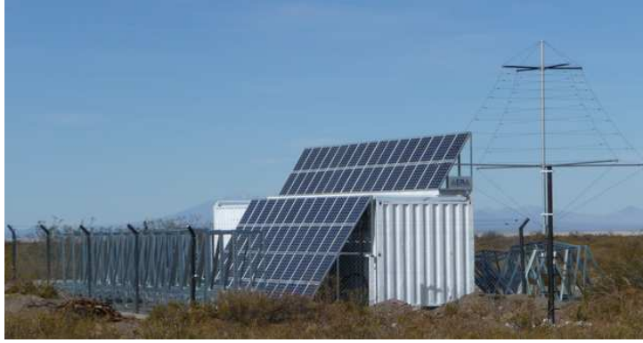
Figure 5.7: The central radio station installed at the AERA site. The CRS serves as central data acquisition to the RDSs. Furthermore, electronics placed in the CRS form the high level trigger of the radio detector. 39 m 2 of solar panels allow an autonomous operation of the station.
