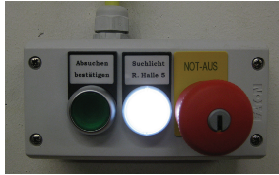
Figure 2: The box including the emergency shutdown button as well as a searching light and an always glowing light for orientation in the dark.
