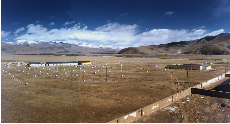
Figure 1.7: Tibet I EAS-PDA at Yangbajing (Tibet). The array consists of 697 scintillation counters (white cubes) spread over a \sim 4 \times 10^4 \text{ m}^2 area at 4 km a.s.l. [177]
