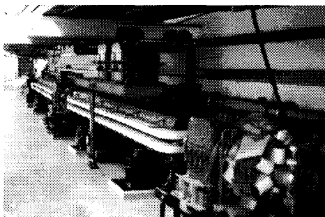
Figure 3 Installation of the first HER arc cell with operating Cu vacuum chamber. A prototype LER raft is mounted above.
