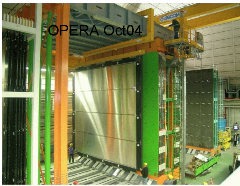
Figure 2.4: Status of detector installation in October 2004. The first magnet is fully installed and the filling of the target modules in the first supermodule had started.
