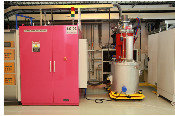
Fig. 4 The modulator and klystron for PAL-XFEL
