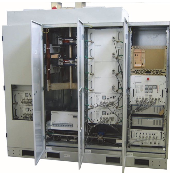
Fig. 11.6. Modular switch-mode 12 kA, 8 V power converter for the LHC.
