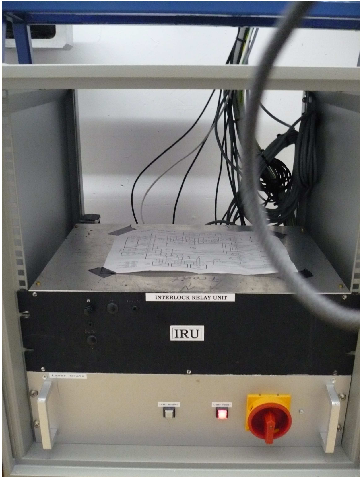
Figure 2.9: Photo of master car power crate.
