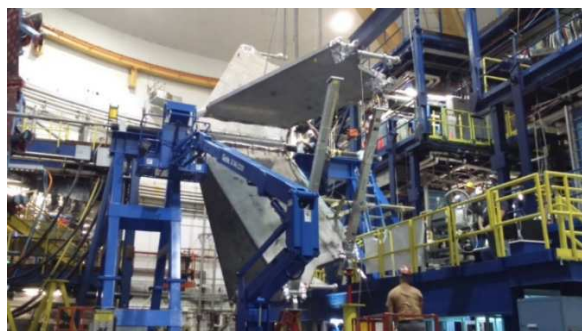
Fig. 8. A coil being “flown” for attachment to the hub and hex beams
