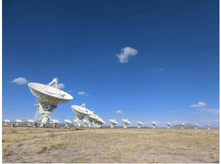
Figure 2.2: Jansky Very Large Array (JVLA, Perley et al., 2011) on the Plains of San Agustin (New Mexico, USA). On Y-shaped tracks, 27 single antennas with a reflector diameters of D = 25 m are connected to operate as a radio interferometer with a maximum extent of 36 km.
